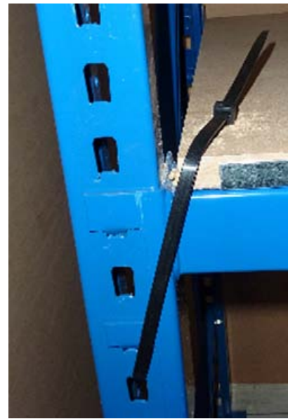
Cable ties hold shelves and shelf rails in place.
